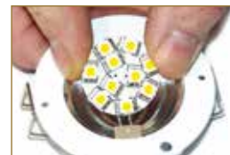
Install the new LuxOr LED
