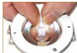
Remove the old bulb
